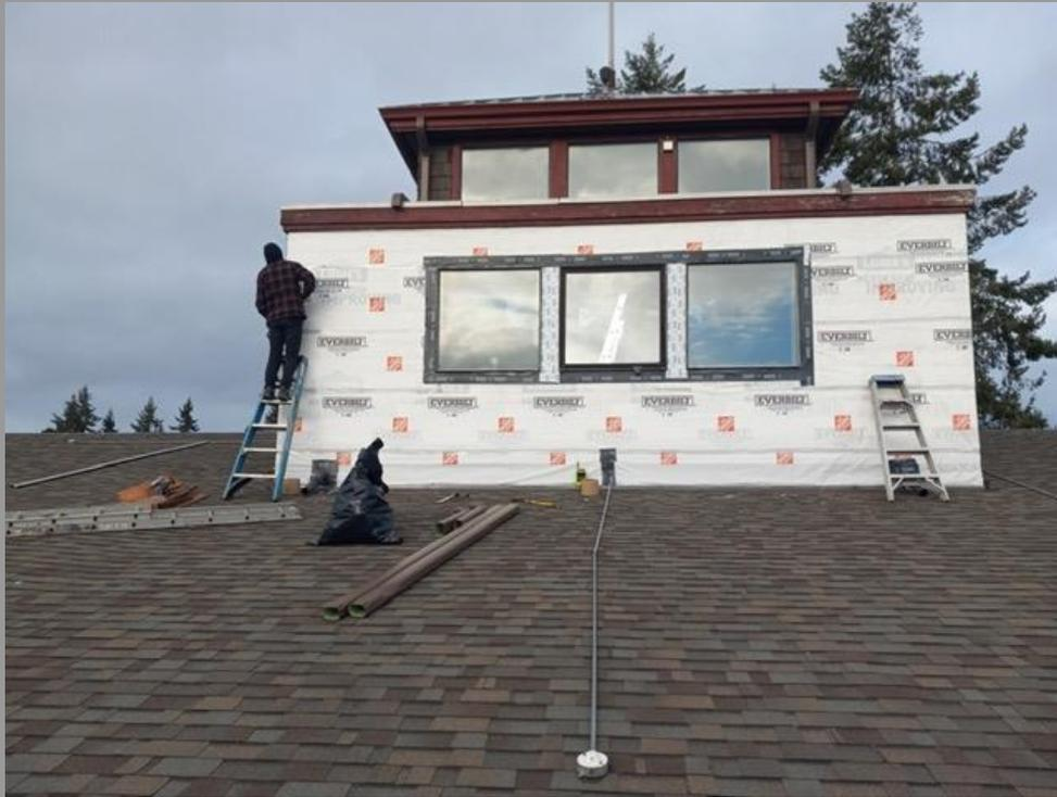
Our wonderful construction contractor, Mark Potter of Poulsbo, has successfully covered the south side of the church lantern and stopped the leaking. These repairs stem from previous work done by Integrity Roofing last year. Once these repairs to the flashing, wrapping, and siding are finished, we can (hopefully) move on to the interior work and resume our regular Sunday services in the Sanctuary. But Mark and his crewmate, Mike, need dry weather to get this done, so pray for sunshine!
